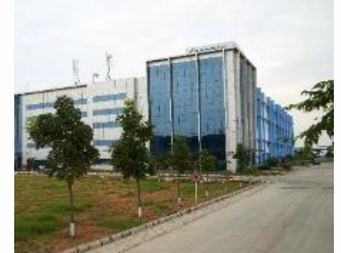
Zero Discharge Facilities
